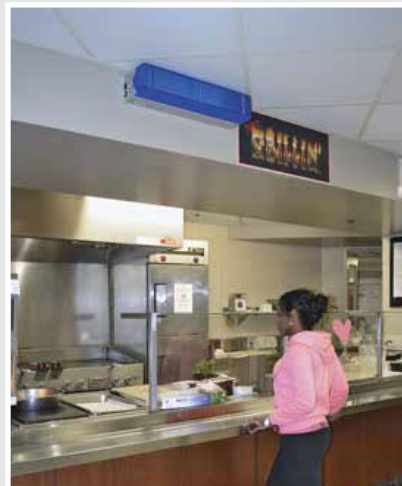
Students order food in the cafeteria as a GLO Upper-Room UV-C fixture disinfects room air.
